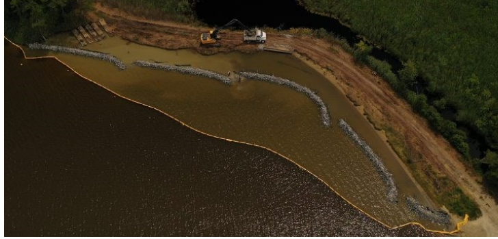
June 2019 Completed toe sills before sand backfill
