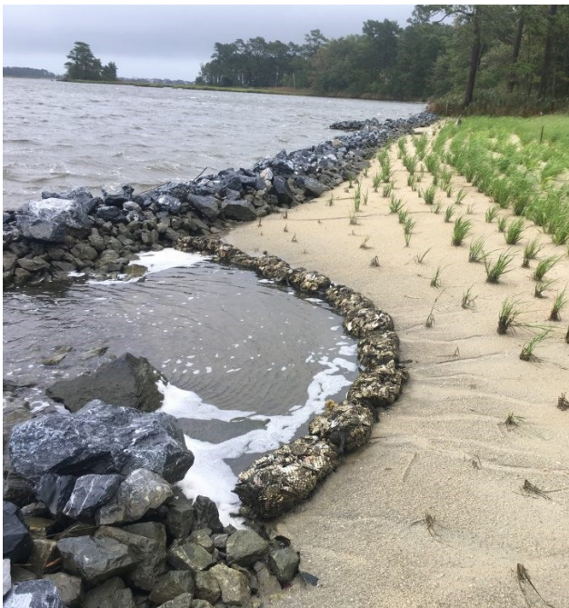
August 2019 Bagged oyster shells stabilizing gap between segments
