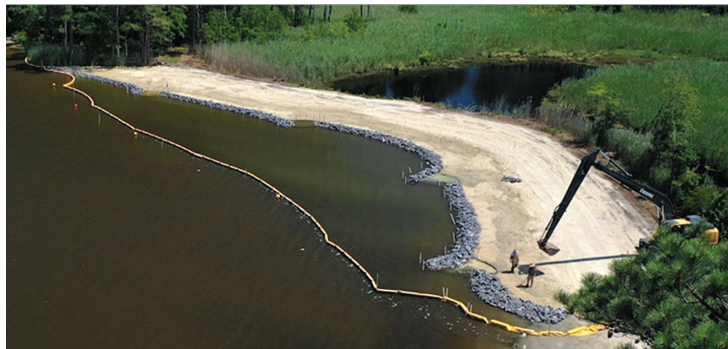
June 2019 Graded shoreline before planting
