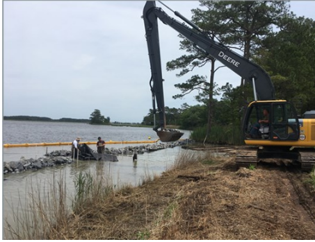
June 2019 Constructing toe sills
