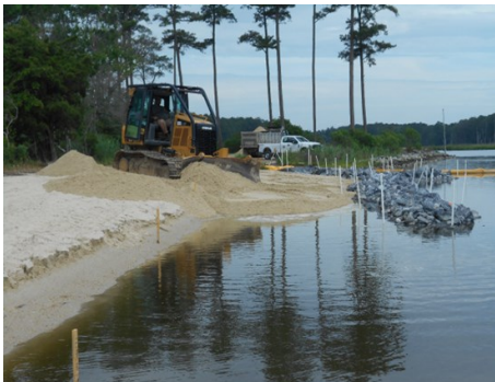
June 2019 Backfilling and grading
