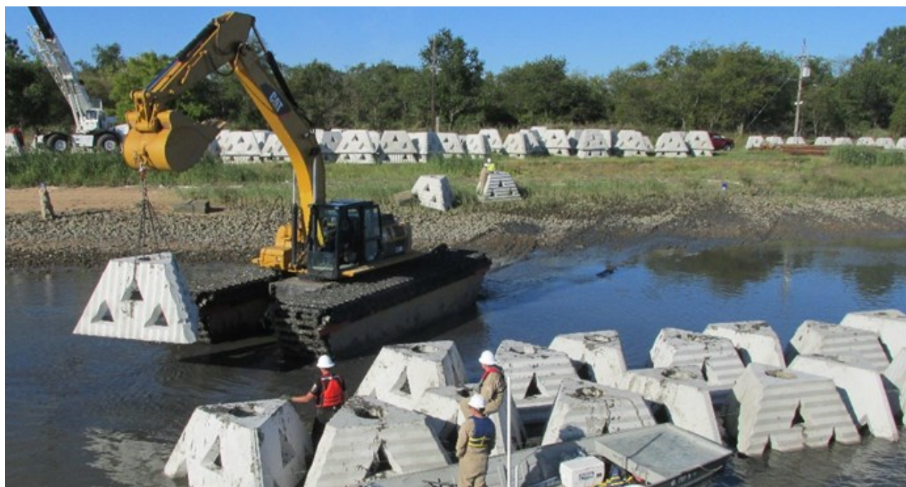
September 2015 Placement of WADs ® with amphibious excavator
