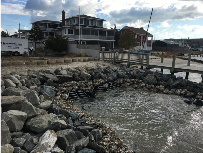
Fall 2019 Completed tide valve assembly
