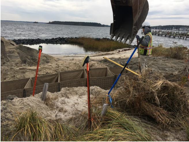
Winter 2019 Hesco barriers installed
