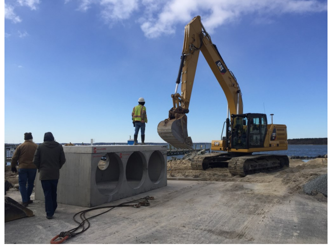
Winter 2019 Box vault installed
